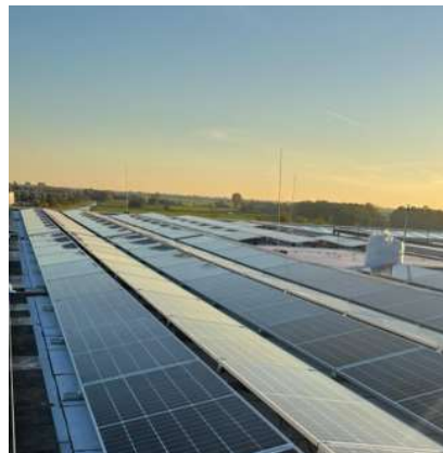
Solar panels on the headquarters in Delft
